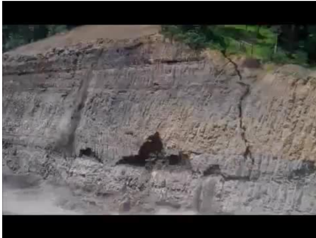
Rockfall during road construction.
